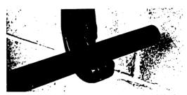
2 Cut the polyethylene tubing square. Tubing should be free of scratches, burrs and cuts. If installation is a service renewal, old steel pipe should be cleaned to prevent scoring of PE tubing.
