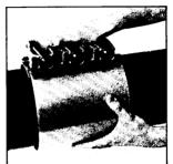
Rotate the clamp in the direction indicated by the arrow to insure proper seating of the gasket, and position the bolts and nuts for convenient tightening.
