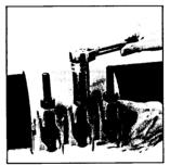
Tighten the bolts working from the center outward. Completely tightening the center bolt will usually stop or sufficiently retard the leakage to simplify completion of the installation.
