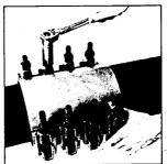
Tighten the bolts working from the center outward. Completely tightening the center bolt will usually stop or sufficiently retard the leakage to simplify completion of the installation.
