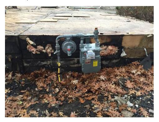
If protective measures are not installed, wind the tracer wire around the riser and terminate it above ground, upstream of any insulators. This will prevent shorting to the meter set.
