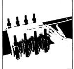
When bolts have been tightened sufficiently to stop the leakage, measure from the reference mark (Instruction 2) to the center of the clamp to see if the clamp is properly positioned over the break or damaged area. Loosen the bolts and reposition the clamp if necessary.
