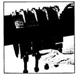
Place the clamp around the pipe centered over the break or damaged area with the gasket flap at the top.
