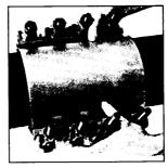
Rotate the clamp in the direction indicated by the arrow to insure proper seating of the gasket, and position the bolts and nuts for convenient tightening.
